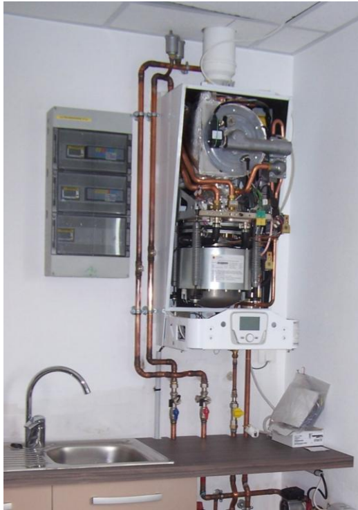
Installation of a mCHP for field test
